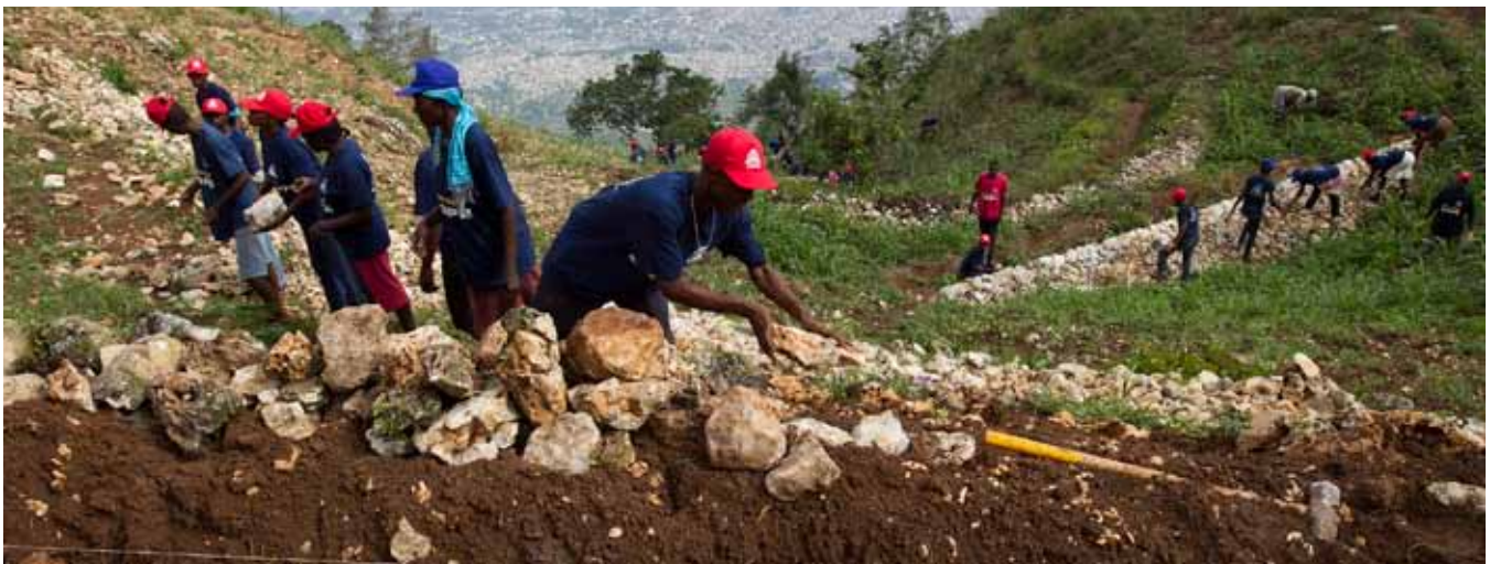
MINUSTAH's Community Violence Reduction program is employing 1,345 local residents in a Cash for Work program building rock walls and planting vegetation as a way of saving arable land and avoiding flooding in lower areas, May 2012. (MINUSTAH/Logan Abassi)
